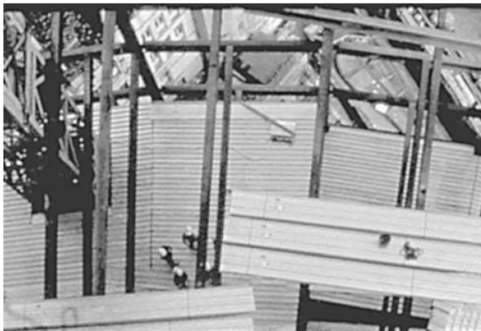
Figure 2.1 Composite Steel-Concrete Floor; Grosvenor Place, Sydney (Uy and Liew 2002)
