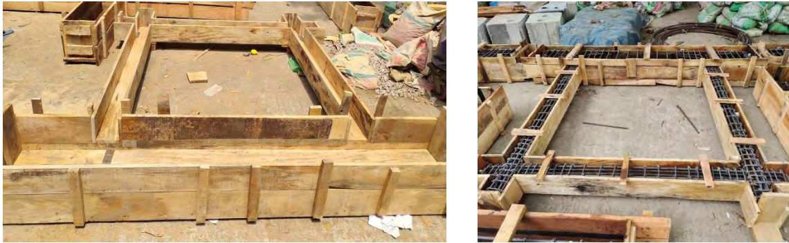
Figure 3.10: Shuttering work.
