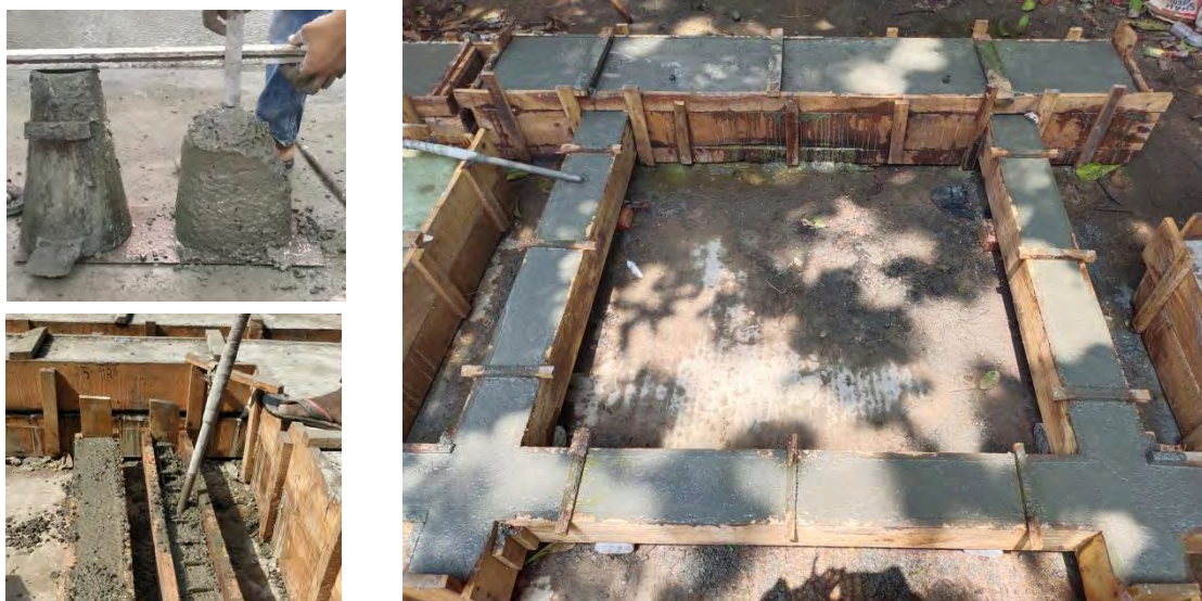
Figure 3.11: Measuring slump and concrete casting.
