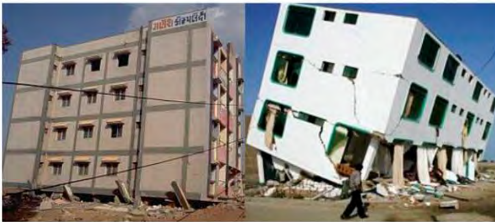
Figure 2.20: Samples of collapses occurred for irregular distribution of infills over the height (Trapani et al., 2015).
