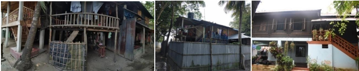
Figure 4.32 Present condition of traditional stilt timber house
