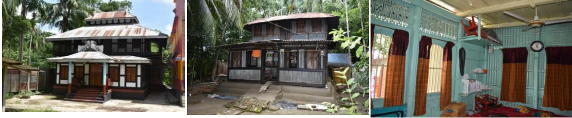
Figure 4.31 Present condition of traditional single/double-storied timber house
