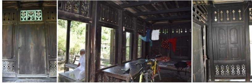
Figure 4.14 Wood carvings for night-time ventilation while windows are kept close
