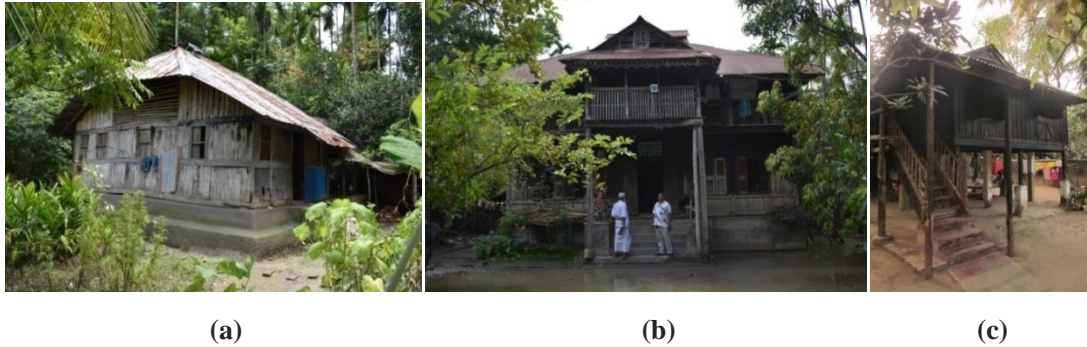
Figure 2.5 Typology of traditional timber house: (a) single-storied, (b) double-storied and (c) stilt (Source: Author (single and double-storied timber house) and Google (stilt timber house))
