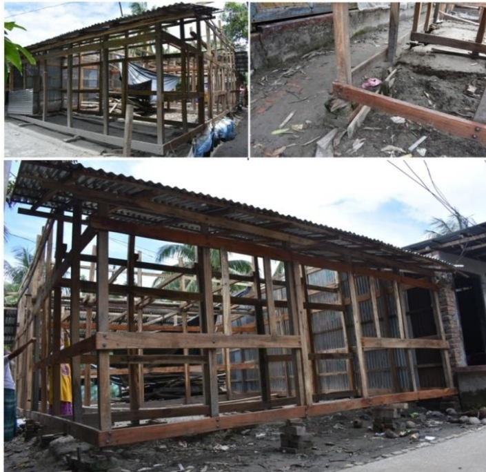
Figure 4.7 Frame structure of traditional single/double-storied timber house
