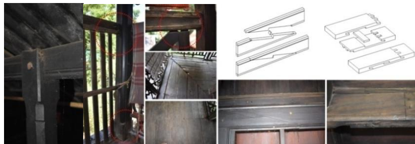
Figure 4.15 Traditional wood joining technique
