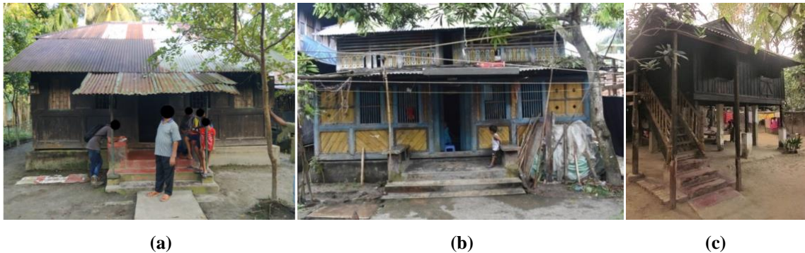
Figure 1.6 Traditional timber houses of Bangladesh: (a) single-storied, (b) Double-storied and (c) Stilt
