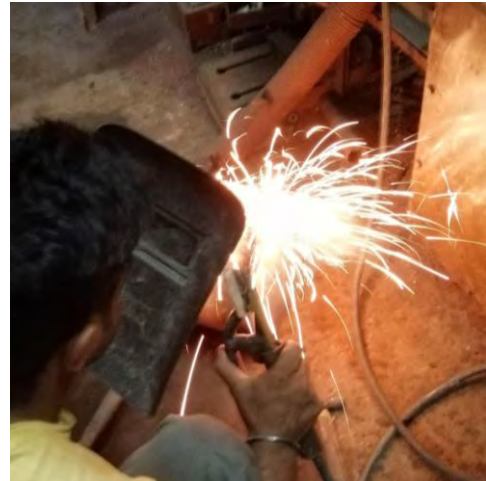
(b) Welding of front MS plate
