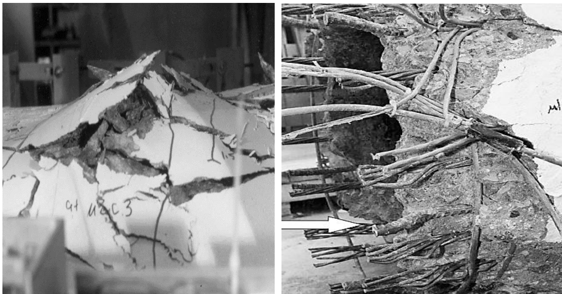
Figure 2.9: (a) Compression failure of hollow pile. (b) Buckled dowel
