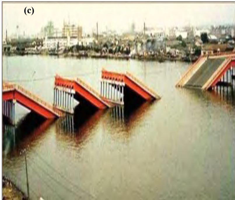
Figure 2.1: a) Lateral spreading Kaushaltar-Lokanthali in Nepal, 2015 (After Gautam et al., 2017) b) Tilting of pile supported building on level ground during 1995 Kobe earthquake in Japan ( After Bhattacharya et al., 2008) and c) The Showa Bridge collapsed during the 1964 Niigata earthquake in Japan (After Bhattacharya et al., 2008)
