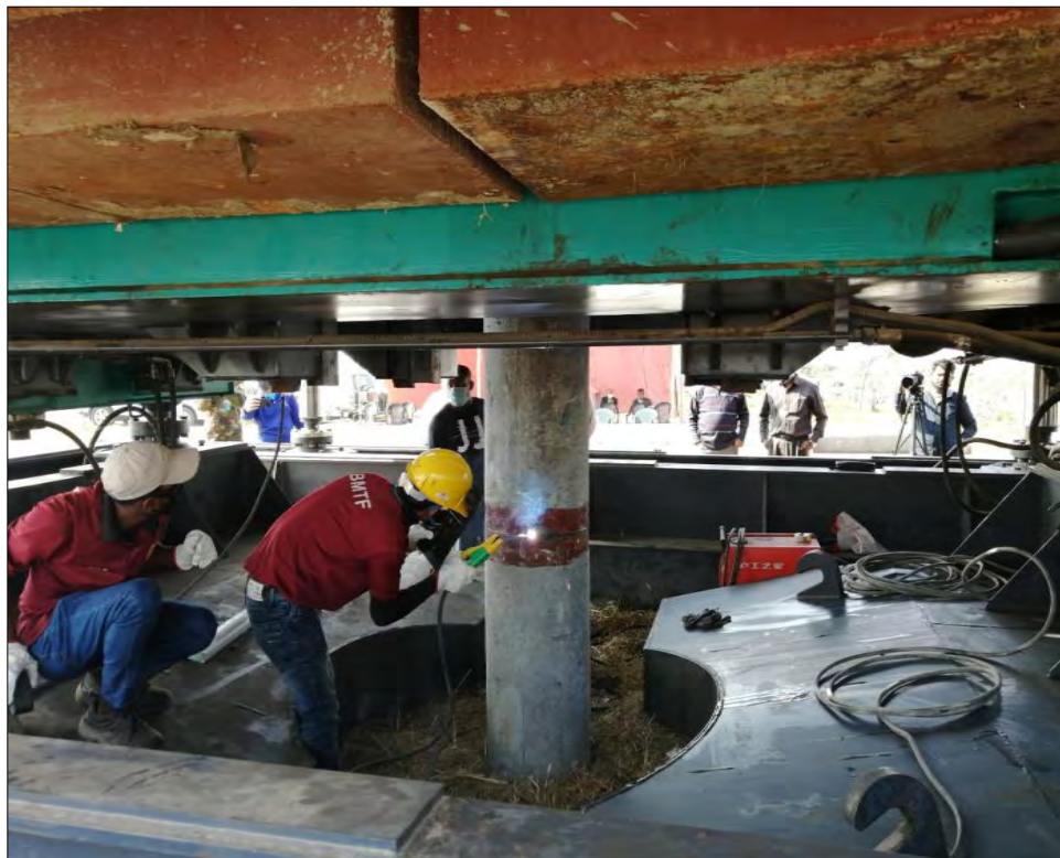
Figure 3.14: Push-in test in study area
