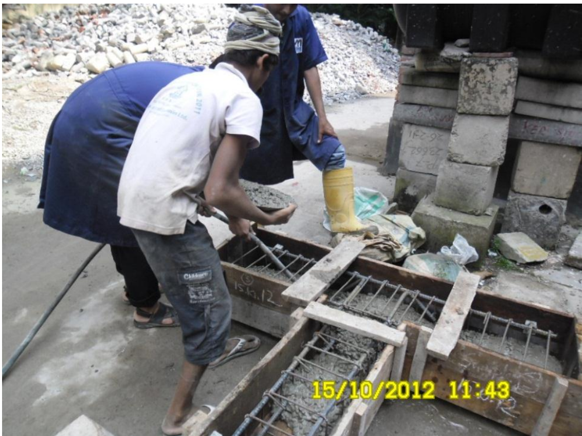
Fig.3.8: Concrete pouring
