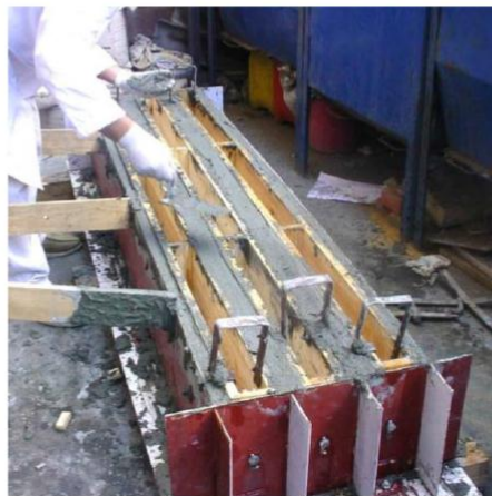
(c) Casting the sides of the U-shaped forms
