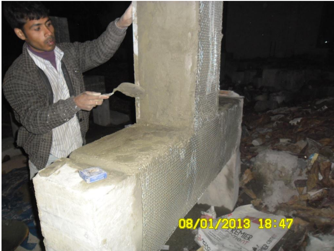
Fig.3.12: Jacketing with ferrocement overlay
