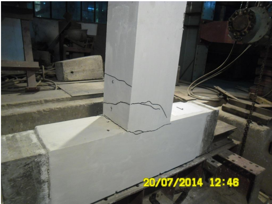
Fig.4.3: After complete failure reference specimen RS1
