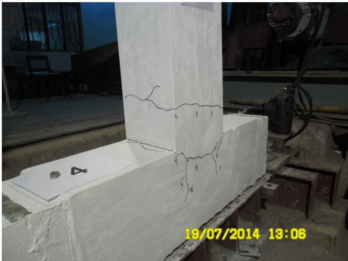
Fig.4.4: Cracking type of failure in reference specimen RS2
