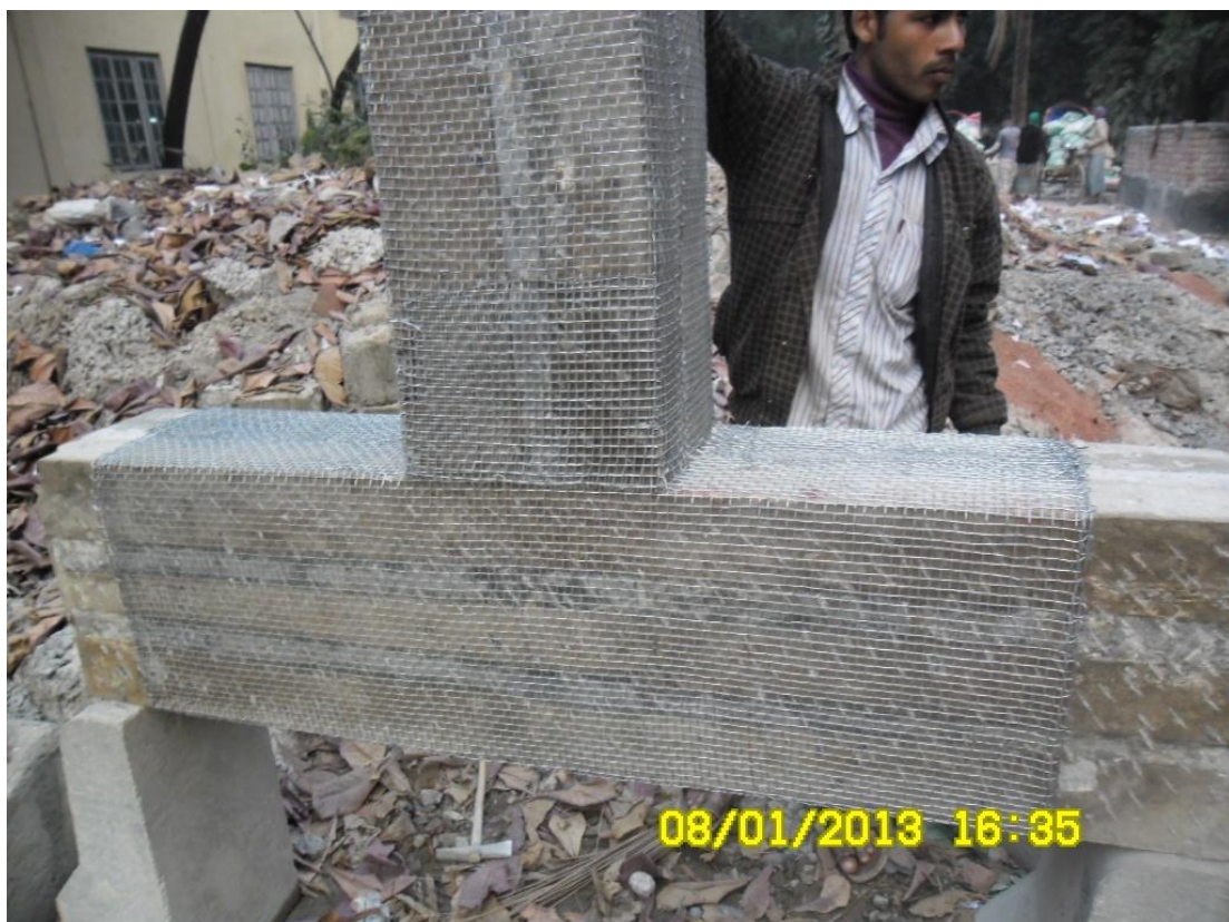
Fig.3.11: Wrapping with wire mesh
