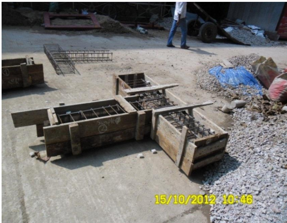
Fig.3.6 Reinforcement placed in the formwork
