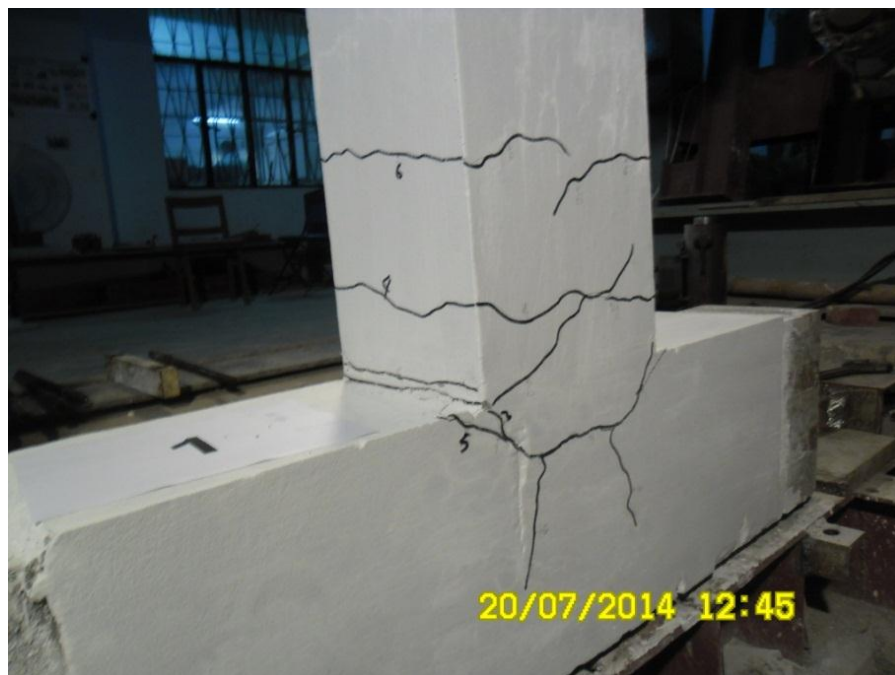
Fig.4.1: Cracking type of failure in reference specimen RS1
