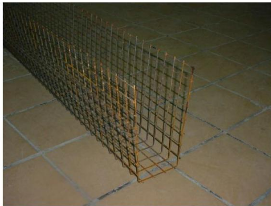
(a) Forming the steel mesh
