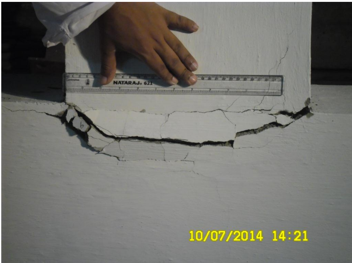
Fig.4.7: After complete failure jacketed specimen JS1
