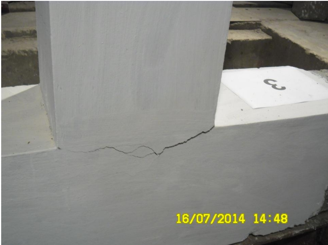
Fig.4.9: After complete failure ferrocement jacketed specimen JS2
