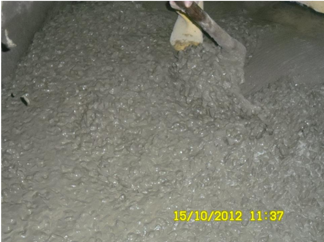
Fig.3.7: Concrete after mixing
