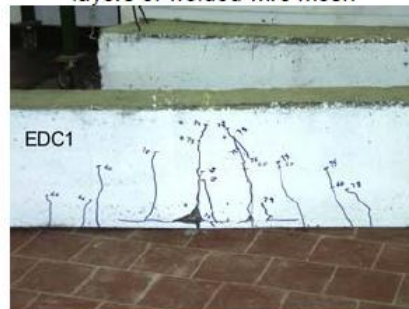
Group 6: Concrete core and double layer of expanded wire mesh
