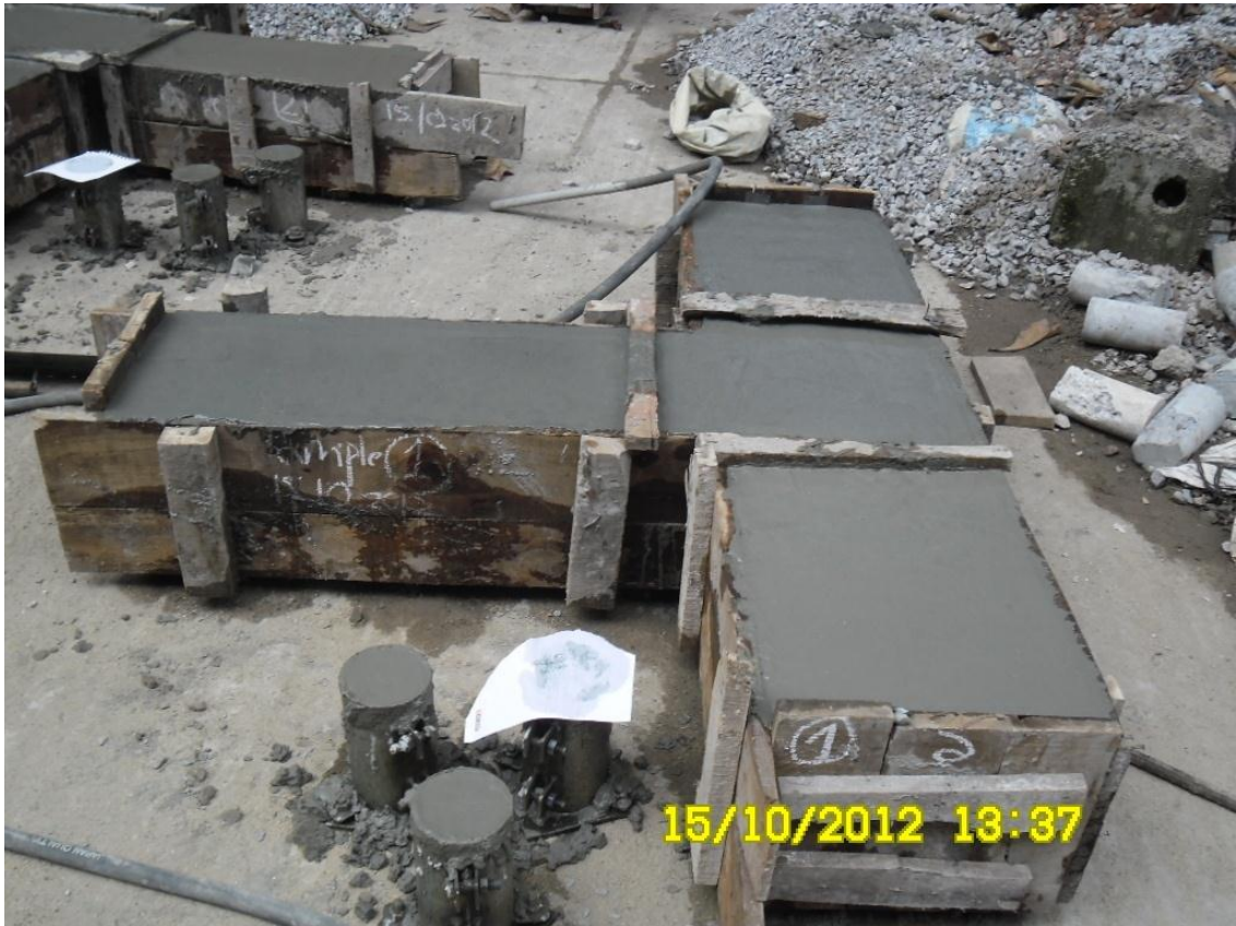
Fig.3.9: Specimen immediate after concreting
