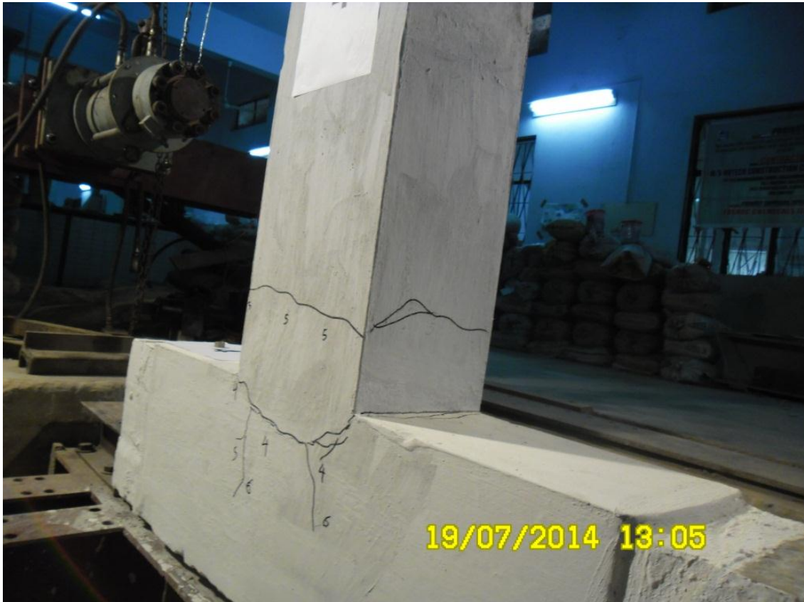
Fig.4.5: After complete failure reference specimen RS2
