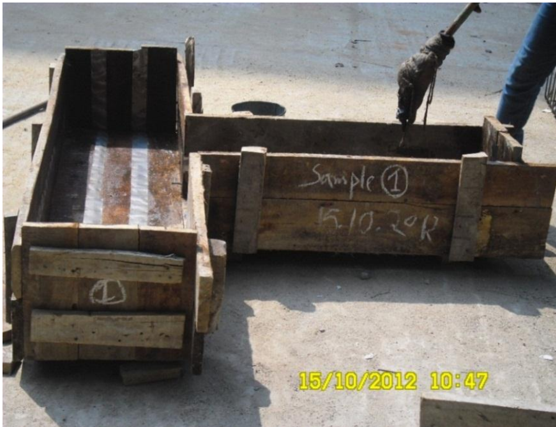
Fig.3.5: Preparation of formwork before concreting
