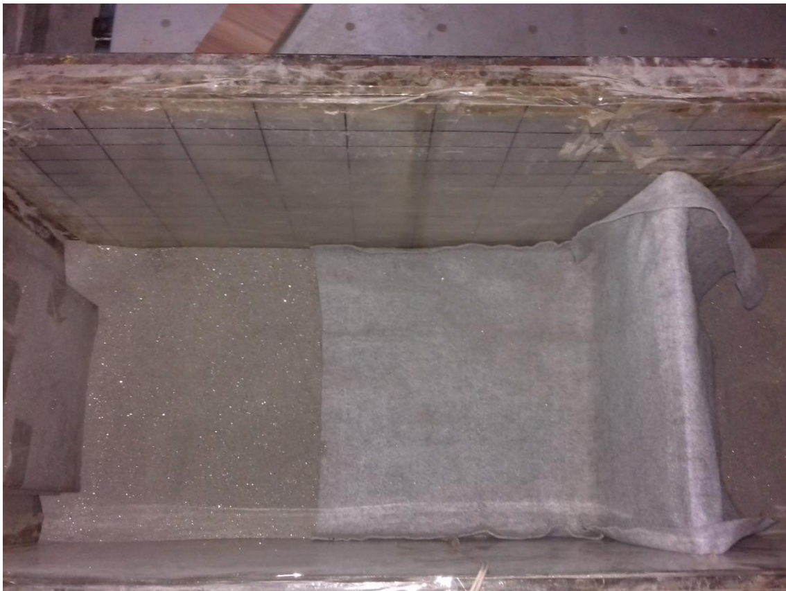
Fig. 3.22 DF50 Geotextile Layer used as Reinforcement
