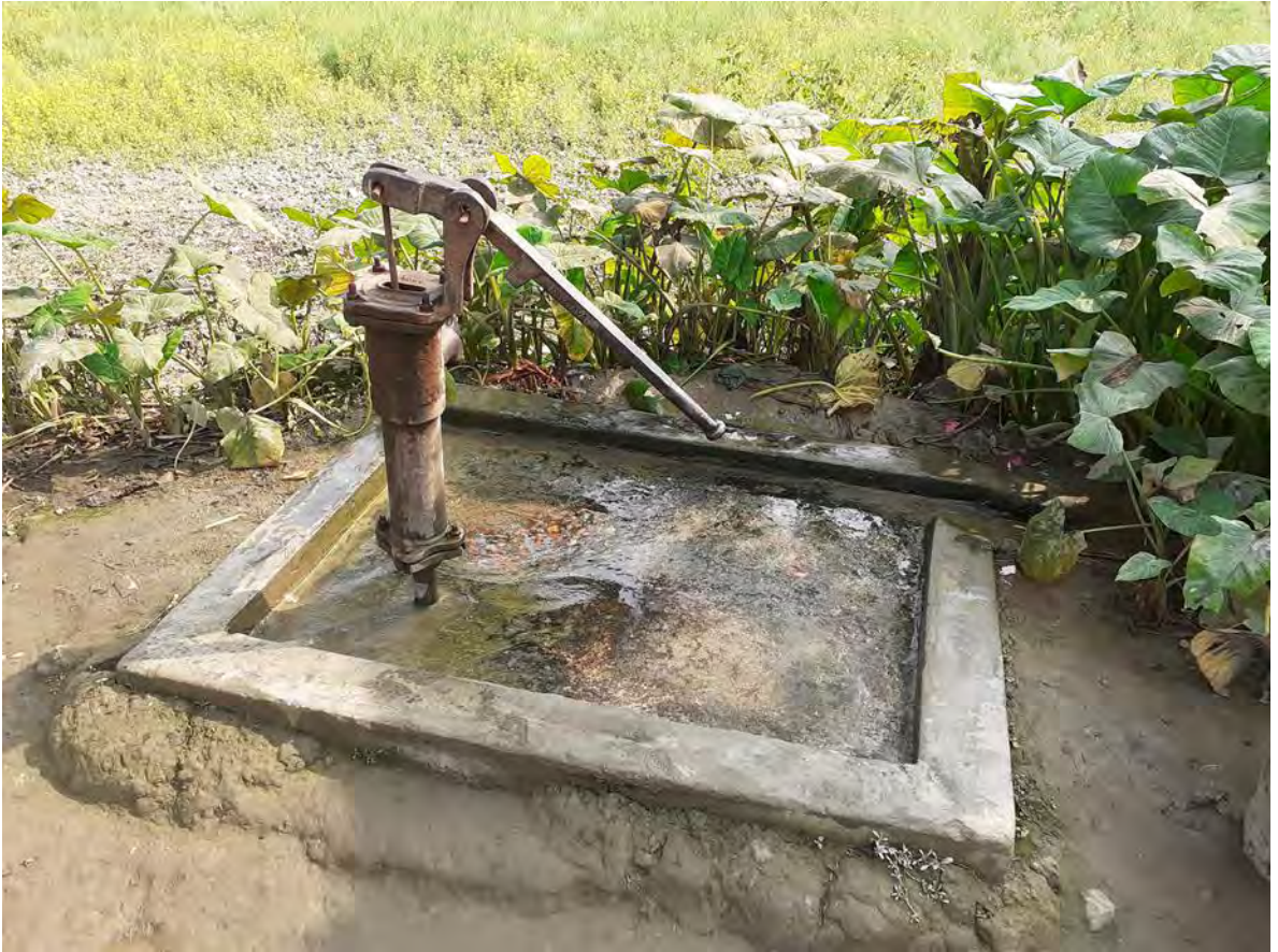
Figure C 23: Drinking water source in Rail line slum
