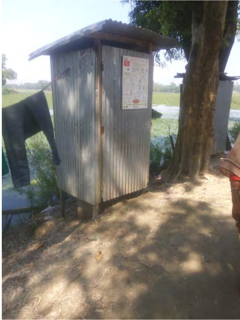
Figure C 12: Sanitation facility in Railline slum
