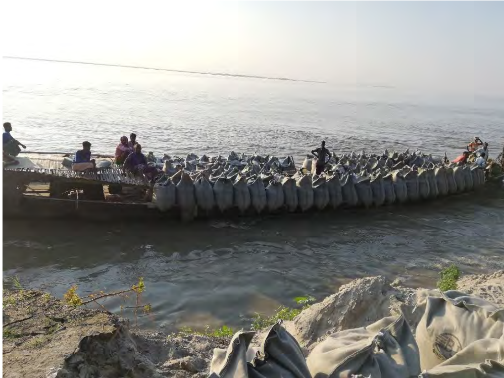
Figure C 9: Ongoing geo bag dumping project of BWDB in Attached Char
