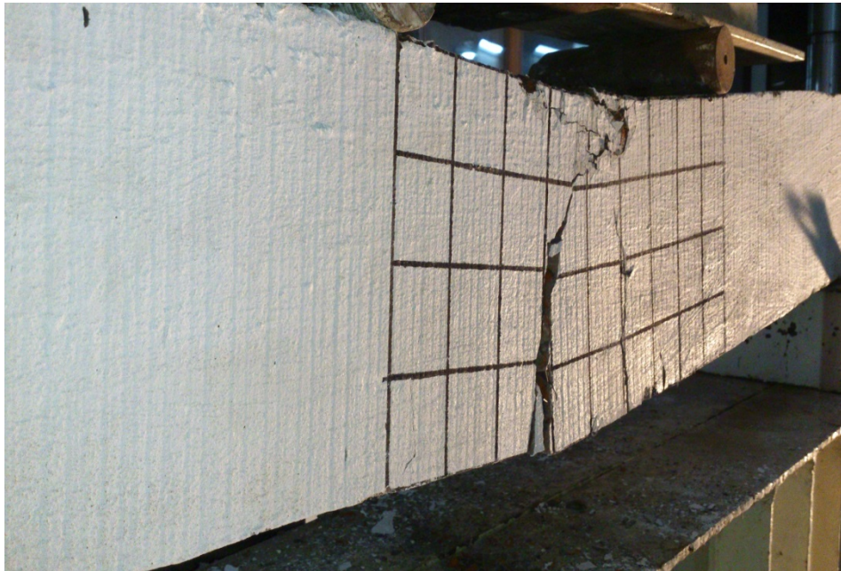
Figure 5.46: Crack-pattern for 2% GWRC specimen
