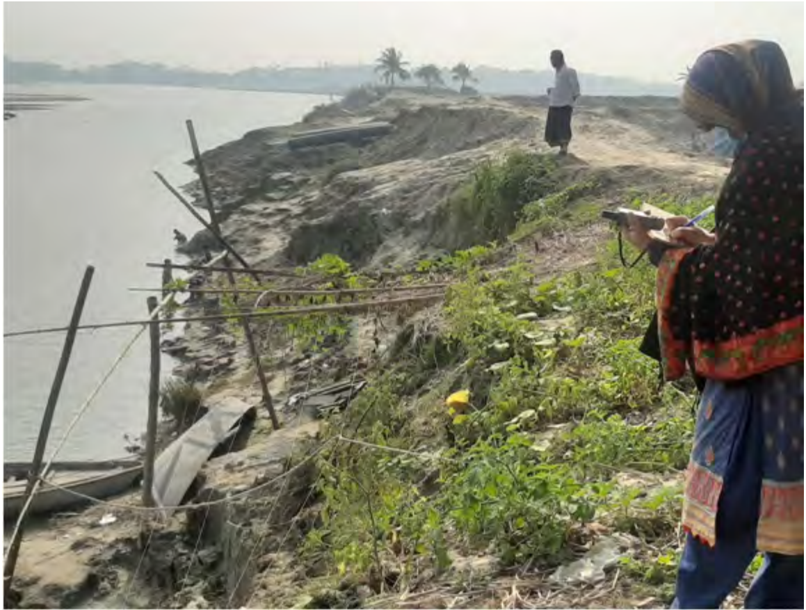
Photo D1: Photo showing location detection by using GPS along the outer bank of the river bend B3.
