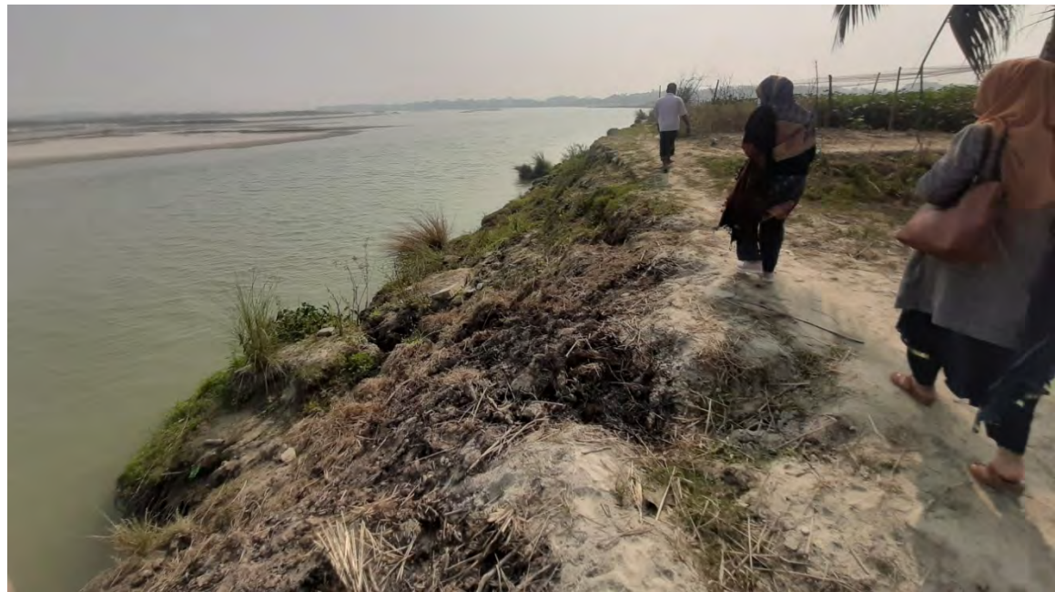
Photo D2: Photo showing insignificant bank erosion at the location of far upstream of the bend apex of the bend B3.
