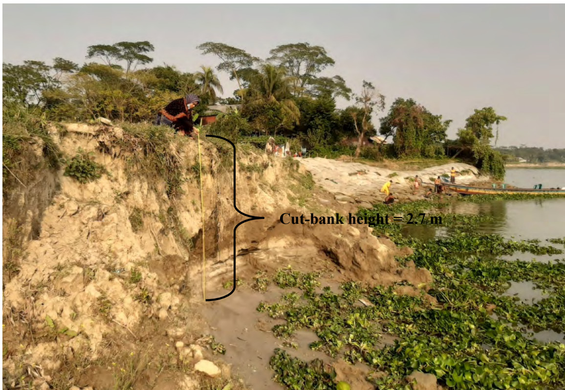
Photo D8: Photo showing the measurement of the height of cut-bank near downstream of bend apex, Bahir Char Katla (N=23°12.055', E =90°14.571') of bend B17.
