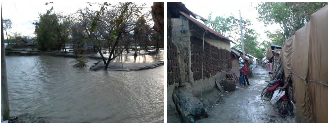
Figure 5.10: Extensive waterlogging insides Polder 29 because of embankment breach, forcing people to live on the embankment
