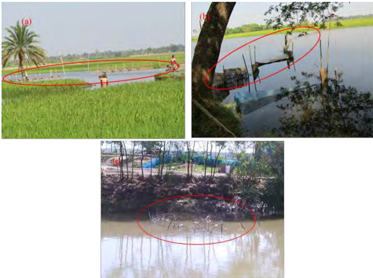
Figure 5.6: Local encroachment in Polder 29 (a) Net (b) Pata
