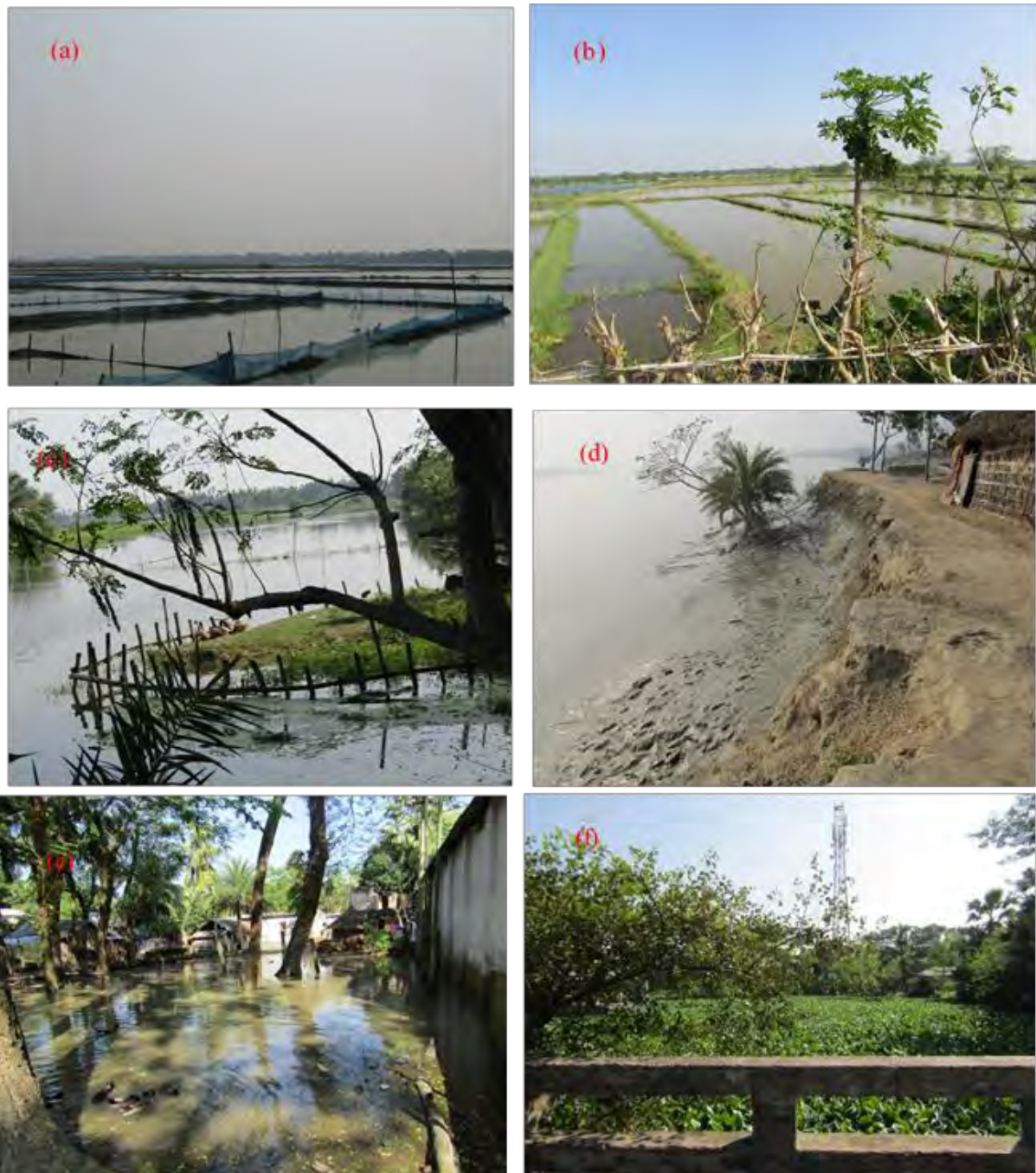
Figure 5.4: Pictures of different issues in Polder 29, (a) Ruhitmara (b) small gher at Bakultal (c) Grabbing khal/river and encroachment for gher at Hazibunia, Telikhali (d) Erosion at Ruhitmara (e) Water congestion, Ratankhali, Bhulbaria (f) water hyacinth blocked canal at Ghona, Kanchannagar
