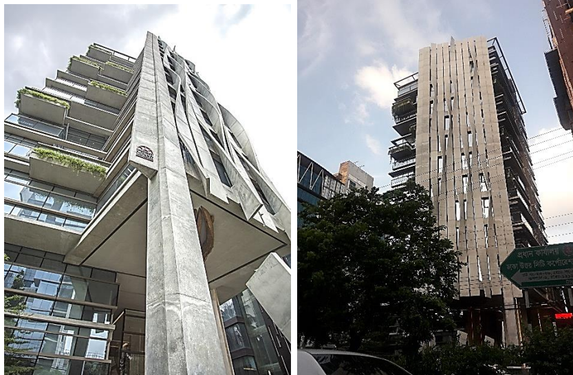
Figure-4.14: Views of South square building (Source: Google Photos and self)
