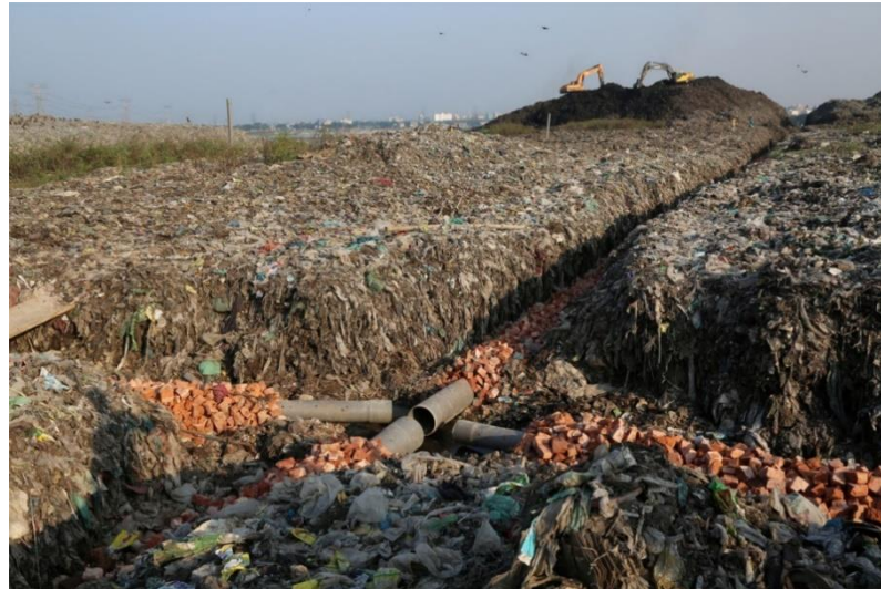
Figure 2.1: Leachate collection system at Matuail landfill (Urme, et al. 2021)
