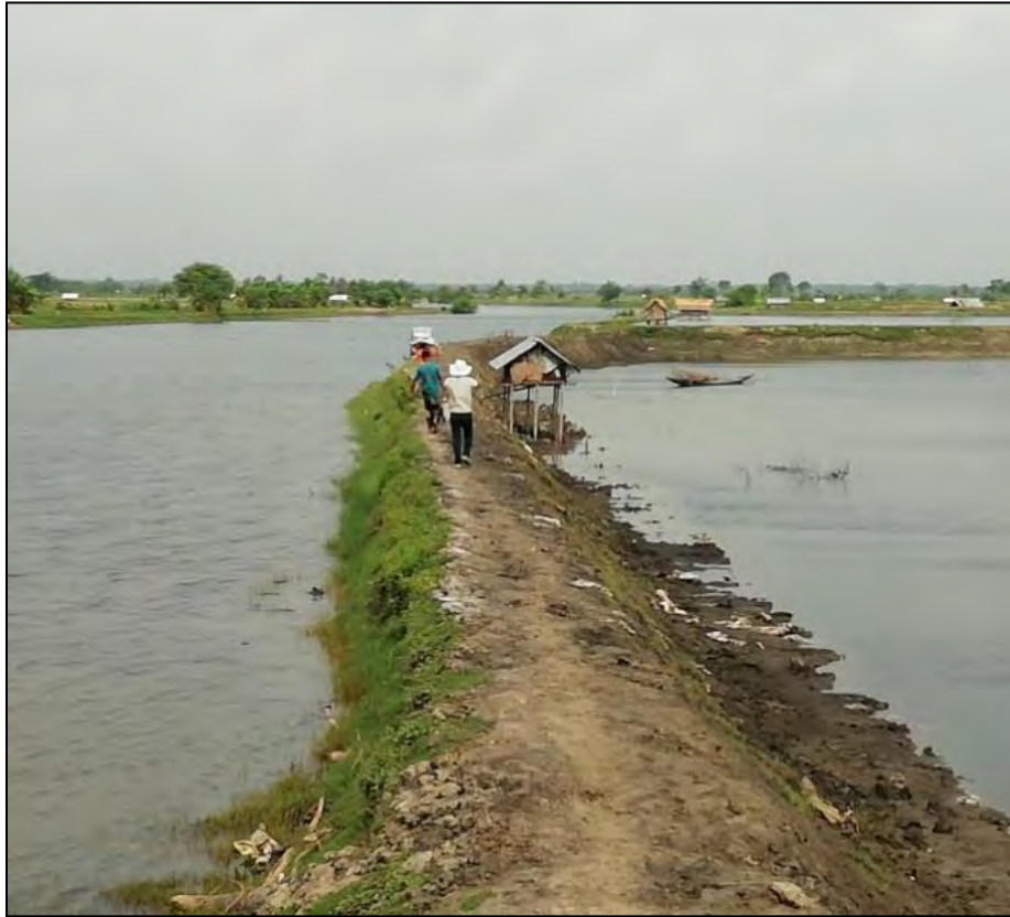
Photo 2.1: A Dike in Beel Bhaina of Polder 24
