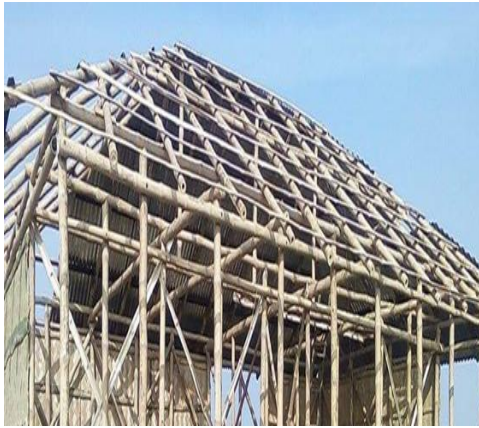
. Figure 6.15: Main & Triangular frame of the roof
