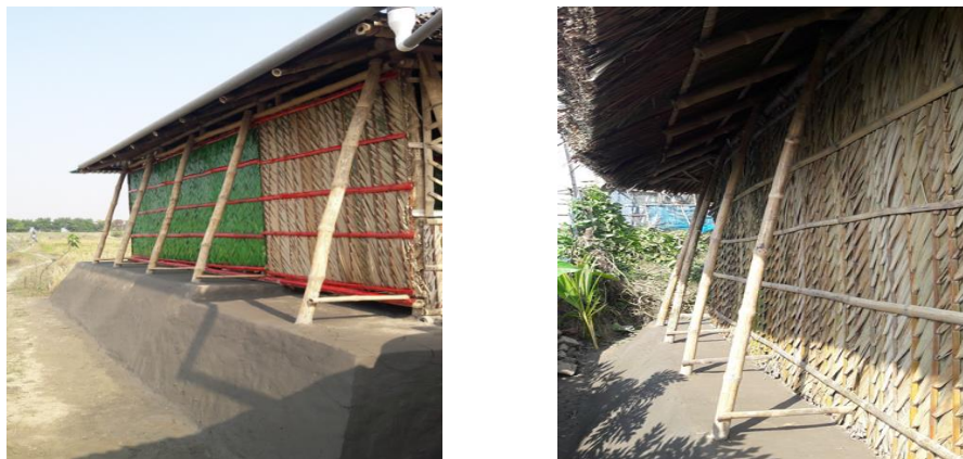
Figure 6.20: Structural buttresses constructed in both implemented design
