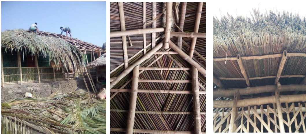
Figure 6.17: Palm leaves thatched installed in the inner portion of the roof to prevent blown off.
