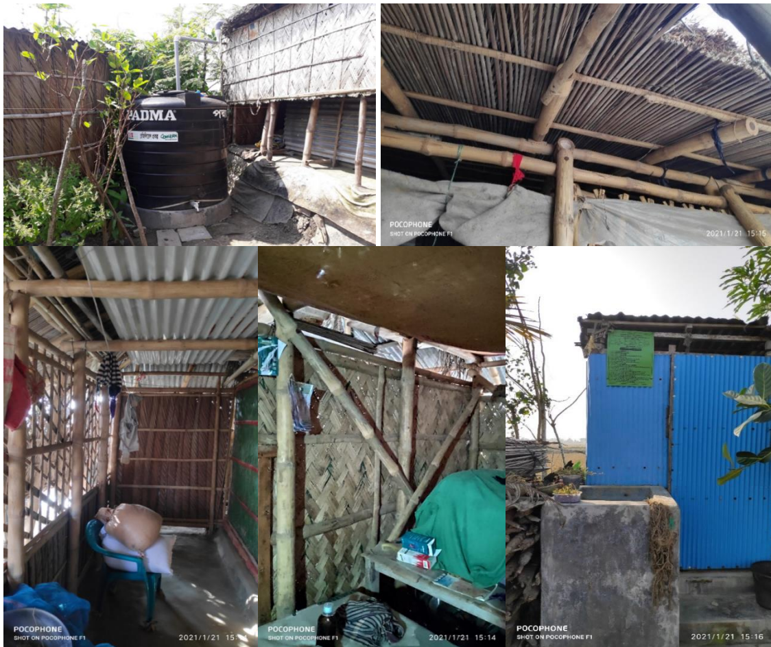
Figure 7.12: Main structure of the designs sustained against impact of four cyclonic events after its implementation. (Captured date: 21.01.2021)
