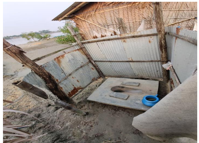
Photo B 8: Sanitation system in Sreenagar village
