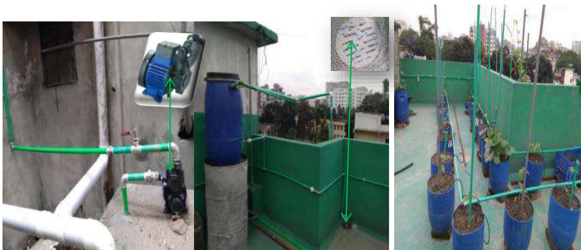
Figure 3.6 Drip Irrigation Setup with Grey and Rainwater Supply in the experimental plot.
