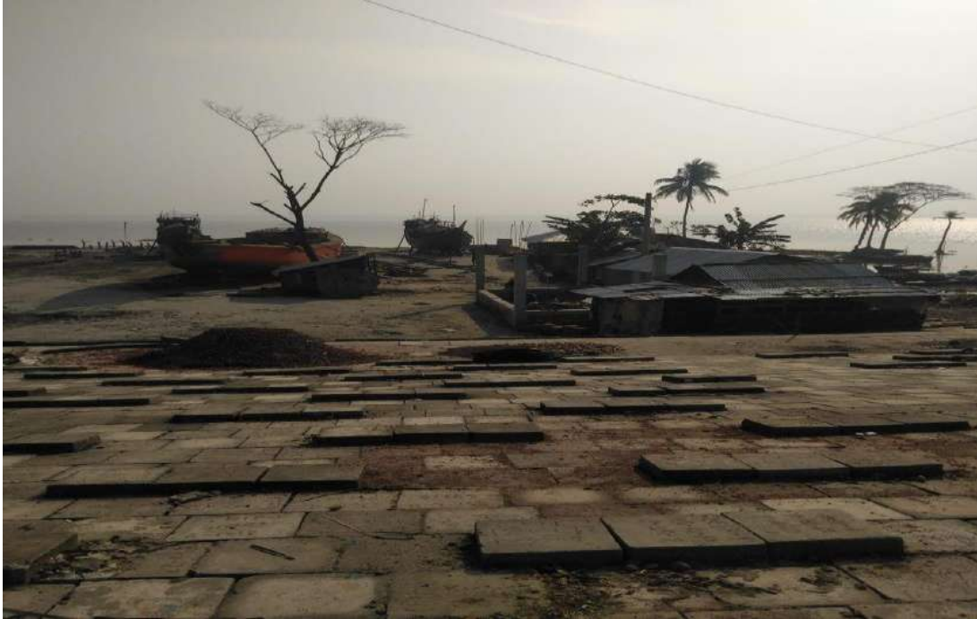
Fig 3.11: Riverbank beside Baleshwar River of Sarankhola
