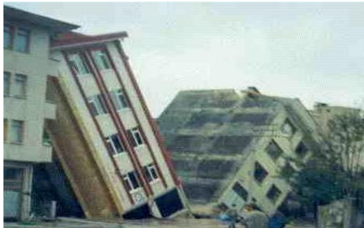
Fig. 2.13 Large deflection in soft story due to earthquake; Bhuj 2001
