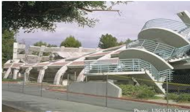
Fig. 2.15 Failure because of the effect of soft story mechanism; Los Angeles, 1994
