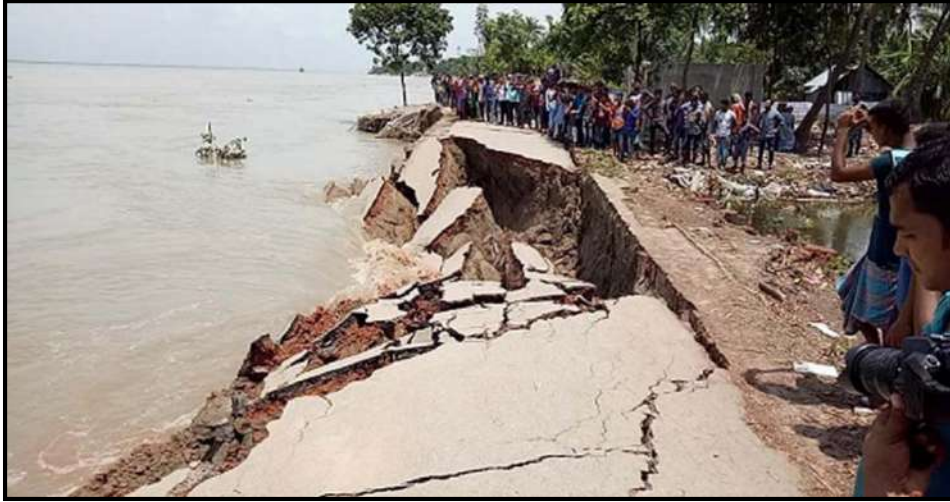
Figure 2.3: Typical mass failure of river bank (Source: Padma erosion in Shariatpur, Dhaka Tribune, 1 st November, 2018)
