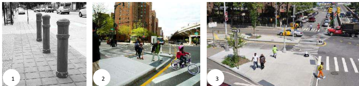
Figure 2.12: 1. Examples of the bollard in Amsterdam (Maas & van Eekelen, 2004), 2. Median cut-through – Nagoya (Iryo-Asano & Alhajyaseen, 2014), 3. Pedestrian refuge island – Hongkong (Saleh, Grigorova, & Elattar, 2020)
