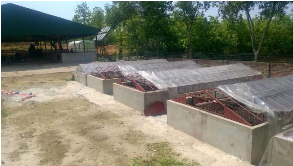
Figure 3.1: Unplanted drying beds at Sakhipur FSTP.
