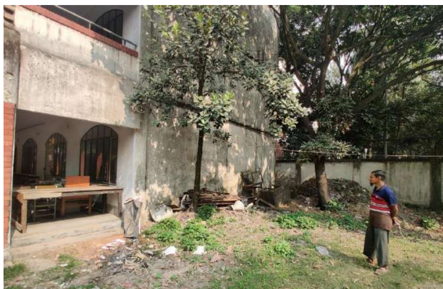
Figure 38 Site before cleaning up.
