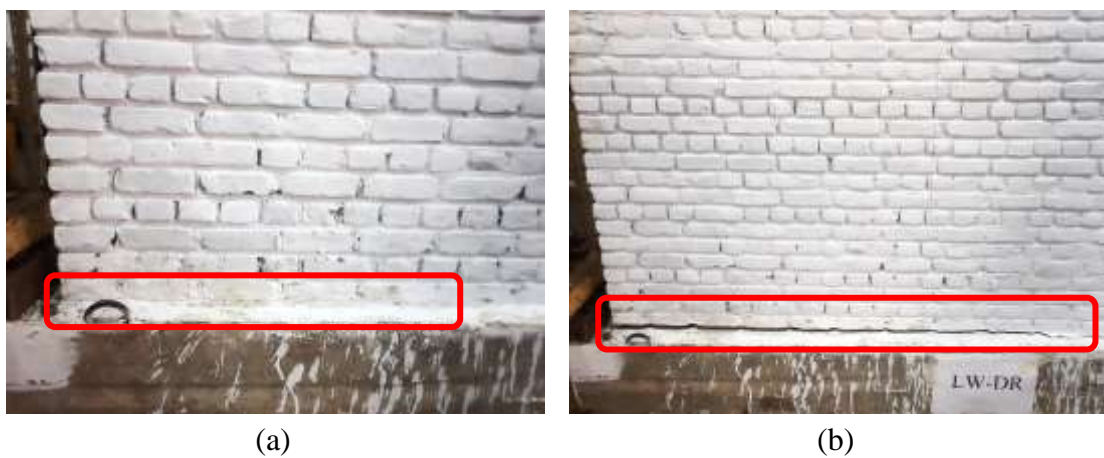
Figure 4.13 Cracks in LW-DR sample: (a) First crack (at base), (b) Final crack
