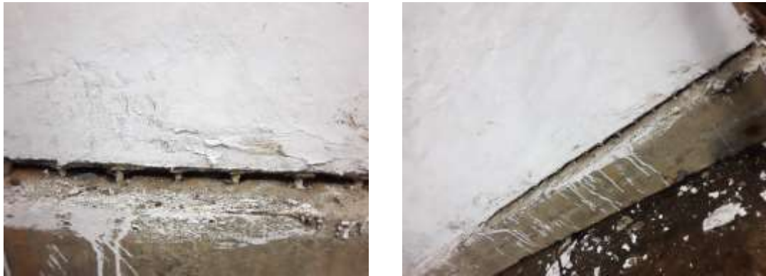
Figure 4.14 Visible rebars of LW-DR after test
