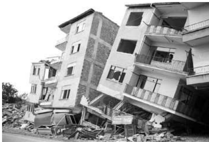
Figure 2.14 Izmit earthquake occurred in 1999 (Turkey) (Yolalmis, 1999)
