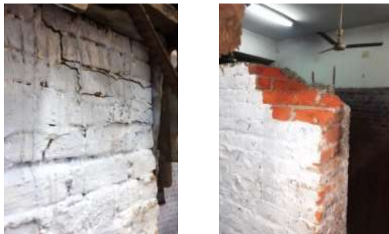
Figure 4.12 Crushing of top corner of LW-CR wall sample
