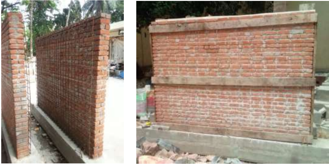
Figure 3.13 Wall sample fully prepared for casting with proper formwork
