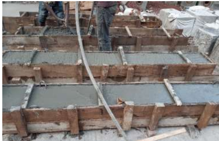
Figure 3.8 Construction of RCC base for masonry wall
