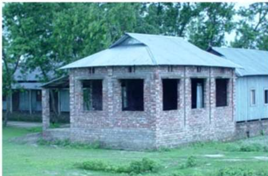
Figure 2.20 Typical Construction of URM Building walls (Ansary, 2003)
