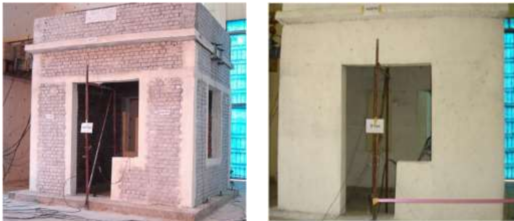
Figure 2.31 Specimen before and after retrofitting (Shah et al., 2017)
