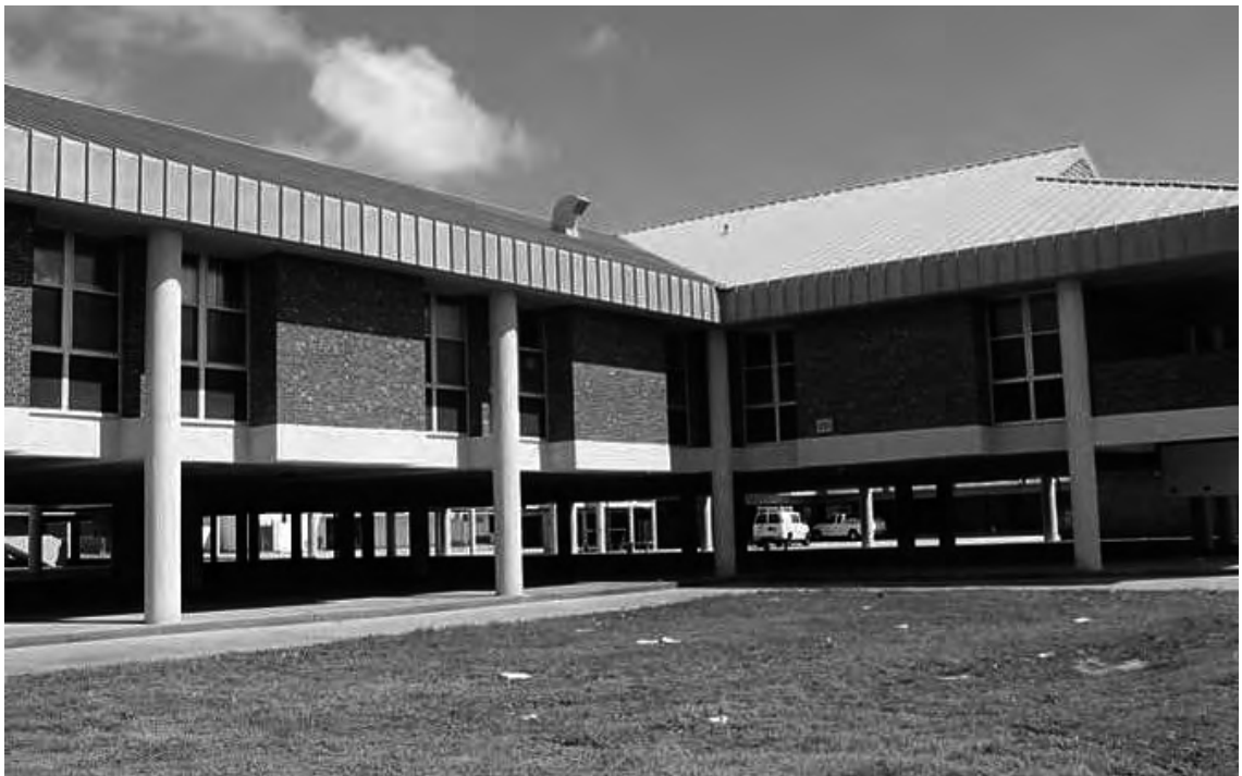
Figure 6.3: School constructed on elevated column to protect from flood
