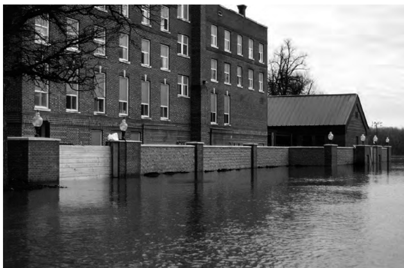
Figure 6.5: Structure surrounded by flood wall to protect from flood
