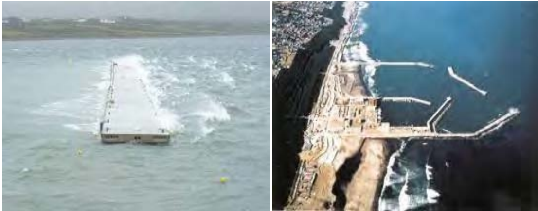
Fig 2.11 shows some photo views of breakwater.
