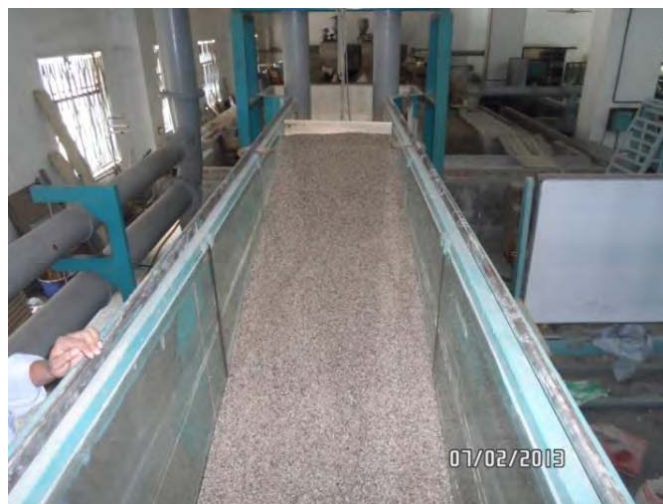
Fig 3.6 stone chips on filter layer.
