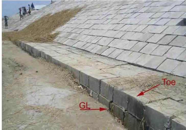
Fig 2.22 C.C. block uniformly place with double layer toe protection.
