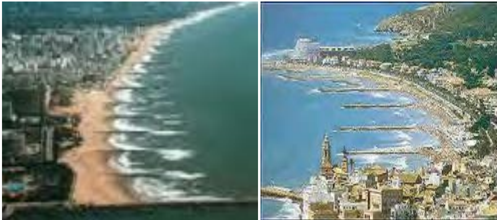
Fig 2.10 shows some photo views of groin.
