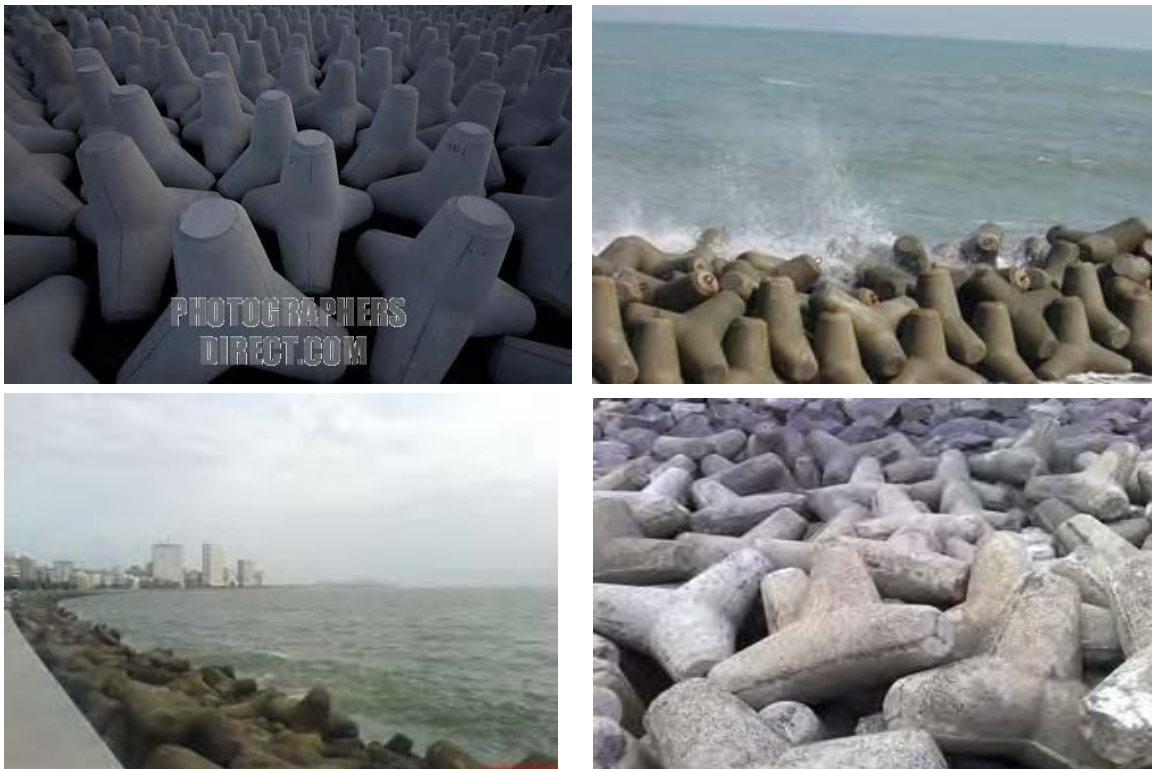
Fig 2.18: Shore protection by Tetrapod.
