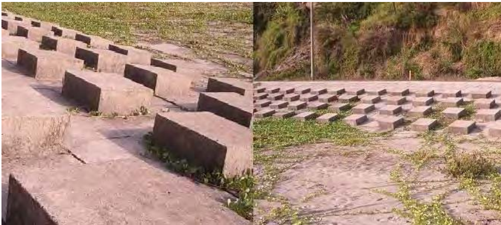
Fig 2.23 Shore protection by C.C. block stagger placement
