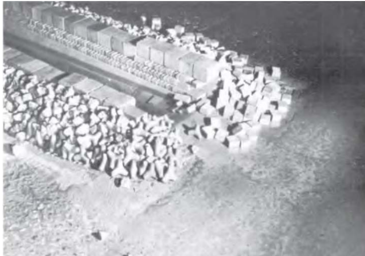
Fig 2.16: Comparative study between a tetrapod mound and classic blocks used for protecting structure.
