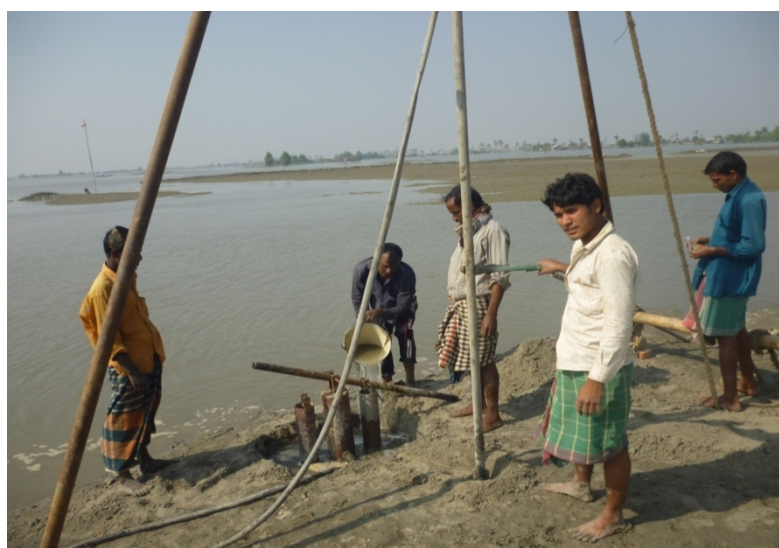
Figure 3.5: Second borehole, BH-1 (15.5 m deep), near new embankment at Patakhali closure, Koyra, Khulna.
