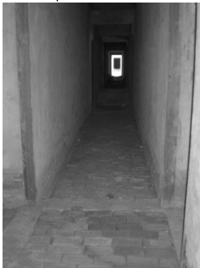
Fig 4.11: Four Feet Wide Double Loaded Corridor
