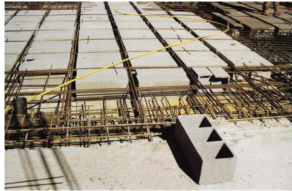
Concrete Hollow Blocks are used on the Roof
