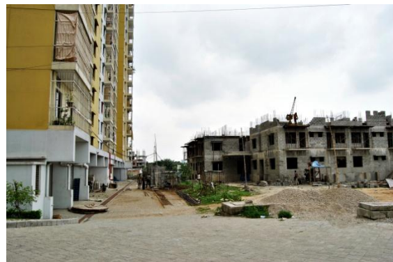
Concrete Hollow Blocks are used in the Wall
