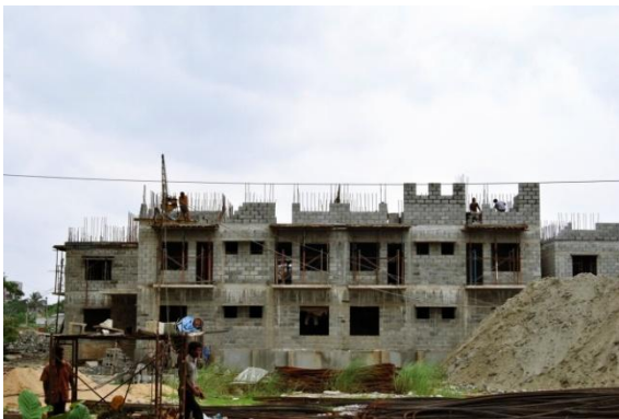
Concrete Hollow Blocks are used in the Wall
