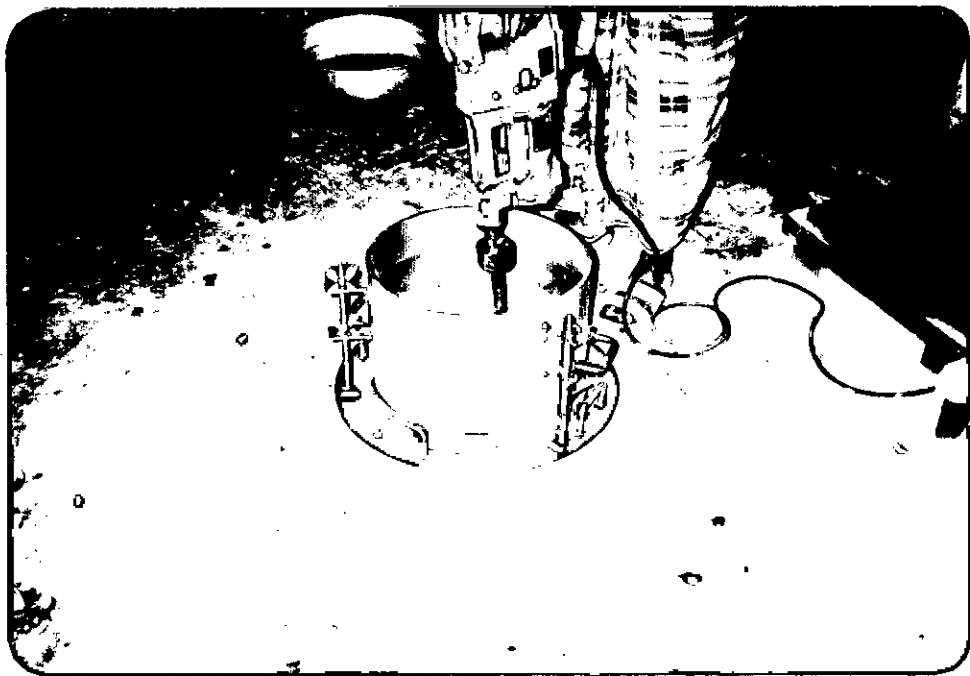
FIG. B-8 COMPACTION OF MBR SAMPLE IS GOING ON BY A BS-VIBRATING HAMMER
