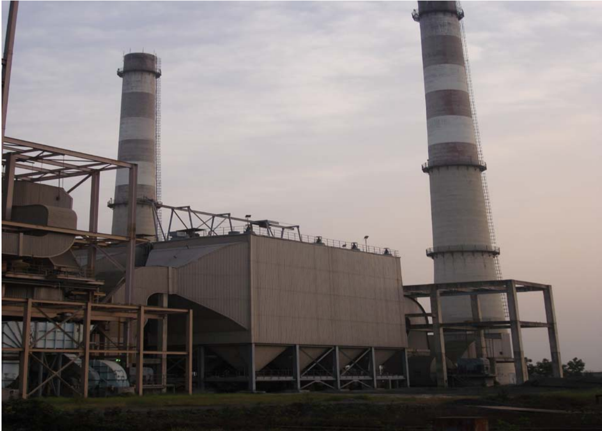
Figure 3.5: Stack of the Power plant
