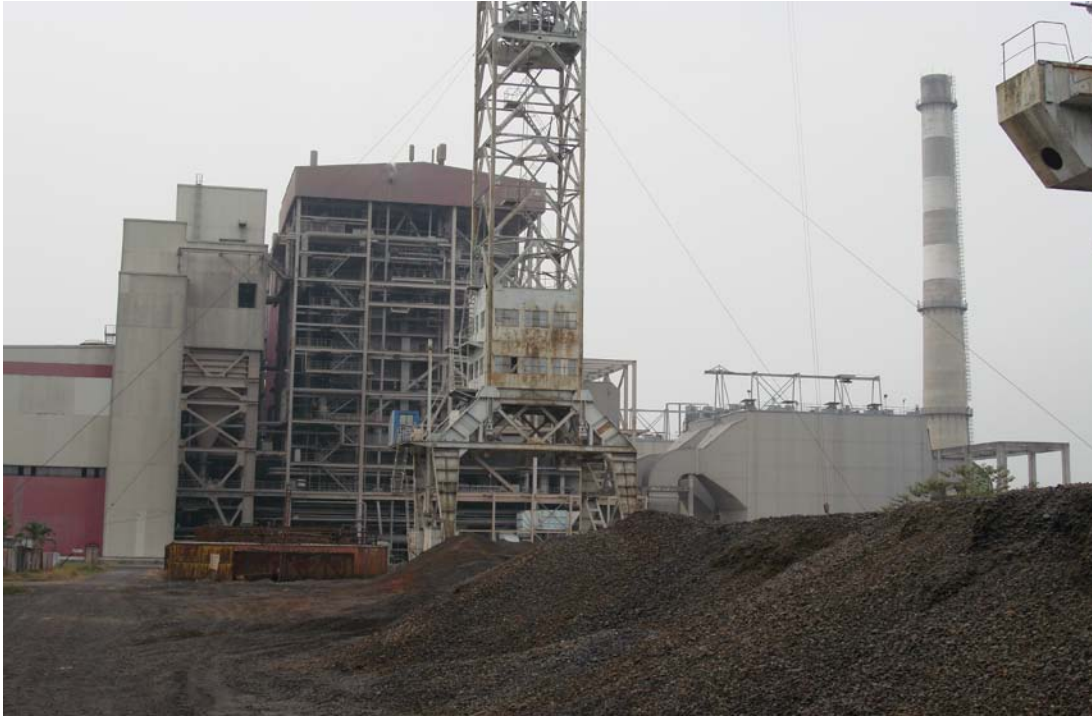
Figure 3.2: Overall view of the Power Plant
