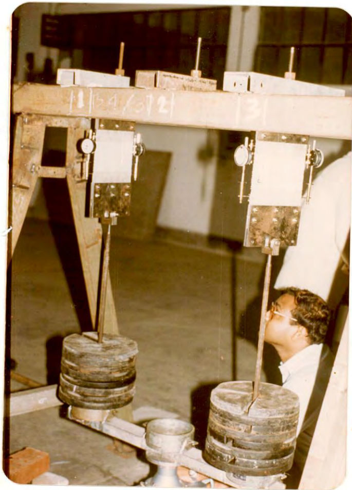
Plate 4.1 Photograph of Repeated Loading Test Rig
