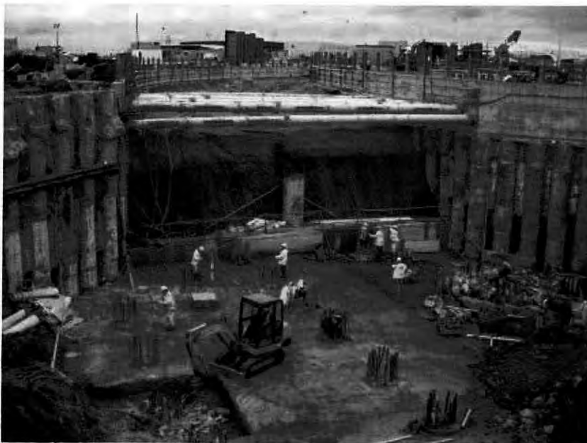
Figure 5.3: Construction of station building (Heathrow ART)
