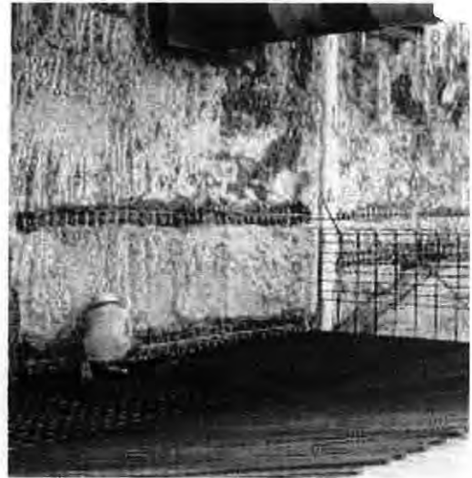
(4) The finished wall after excavation
