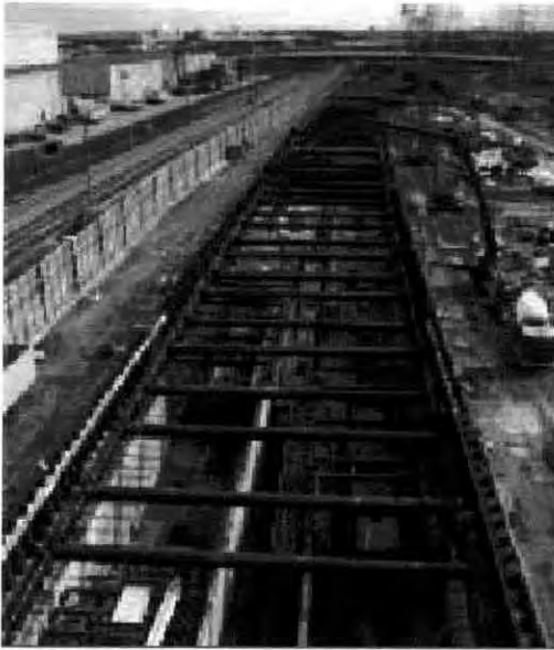
(1) Steel pipes used as struts (Twine D, 2004)
