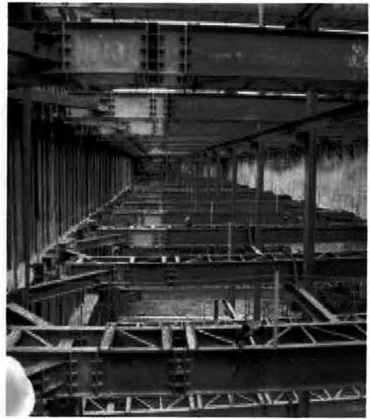
(2) I-sections used as struts (Paya Lebar expressway)
