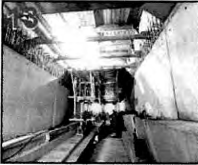
(9) Walls are poured using formwork
