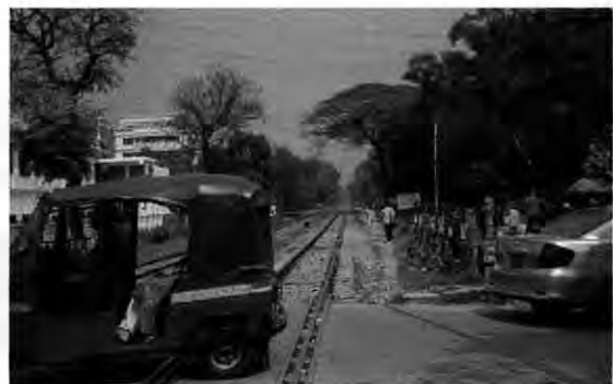
(b) Banani Rail line Crossing
