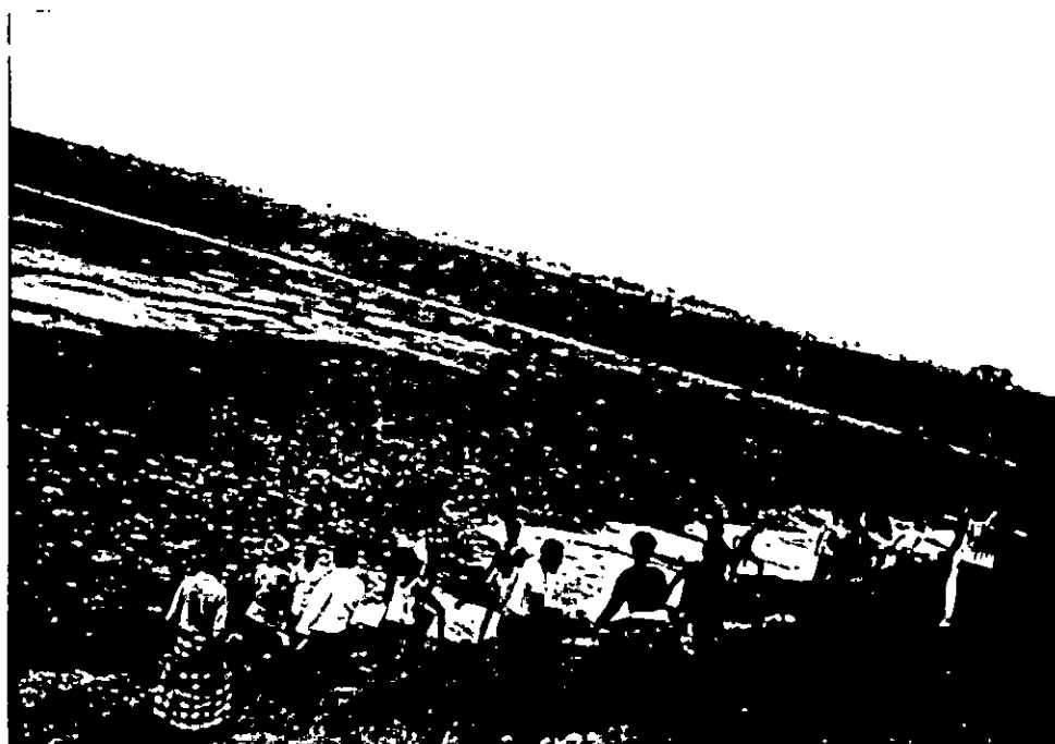
Plate 3.7 Removing of Sludge Manually from Pegla Lagoon
