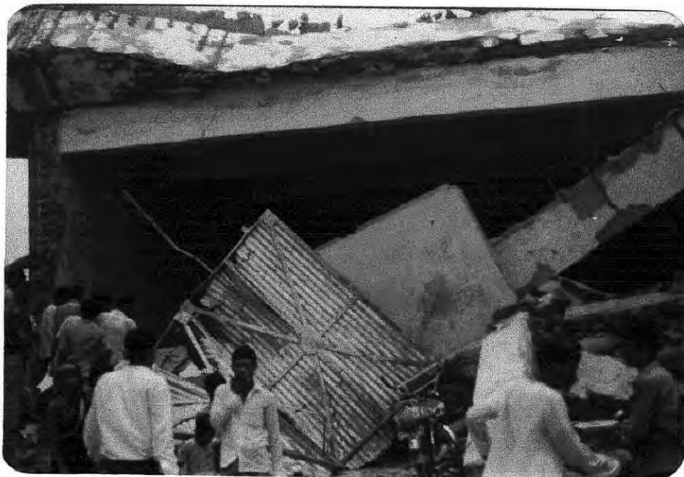
Photo of Damage House Casualty
