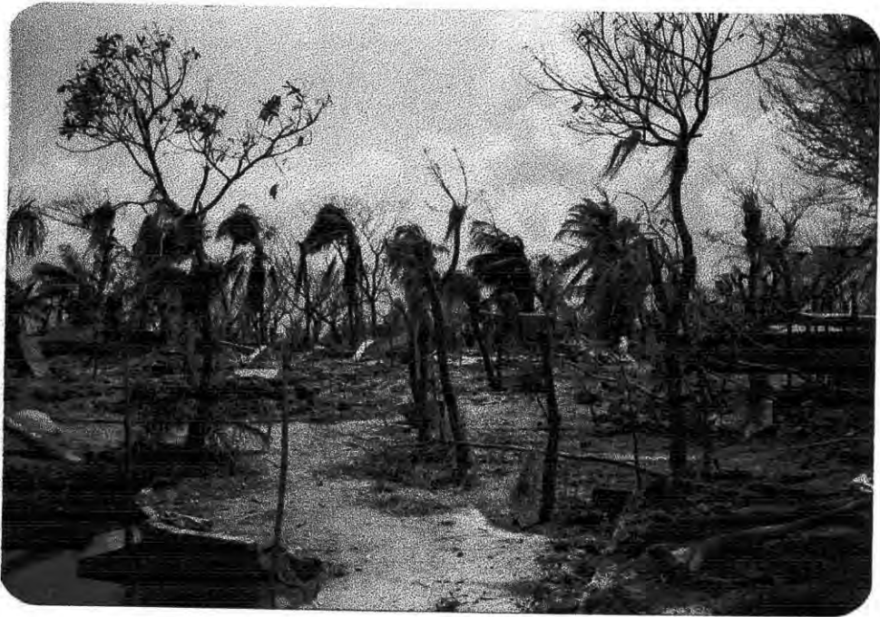
Photo of Damages of Cyclone 1991
