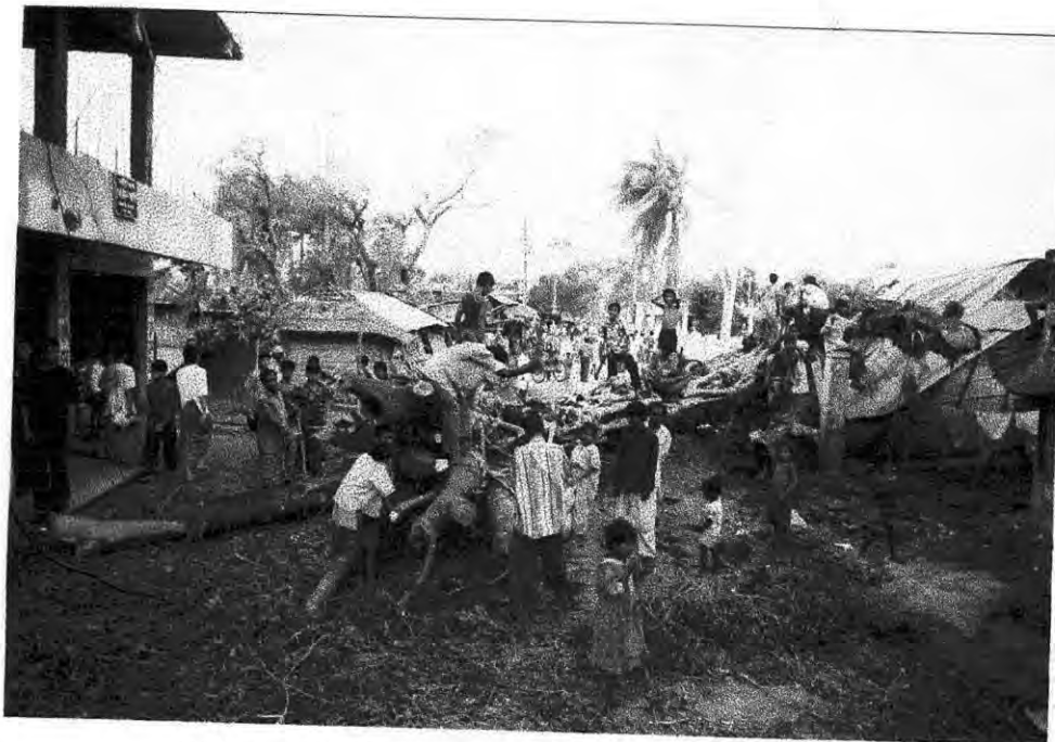
Photo of Damages of Cyclone 1991
