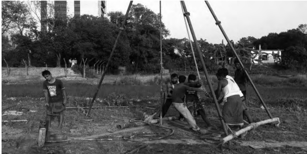
Figure 3.3 SPT Test at MIST.
