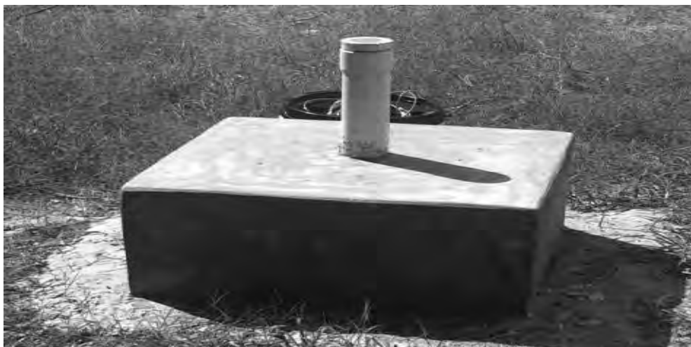
Figure 3.5 PVC pipe cased borehole on the testing location on west side of BUET JIDPUS, BUET.
